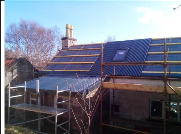
Repair of the roof © Isle Martin Trust
