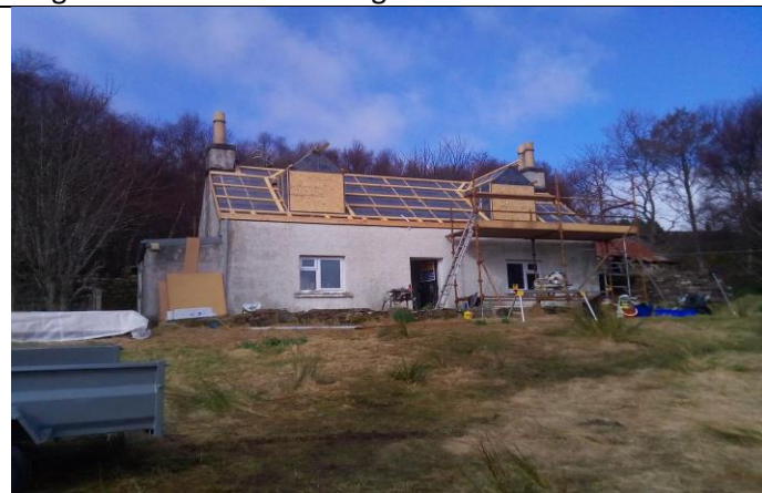
Repair of the roof © Isle Martin Trust
