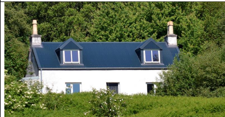
Roof following repair © Isle Martin Trust
