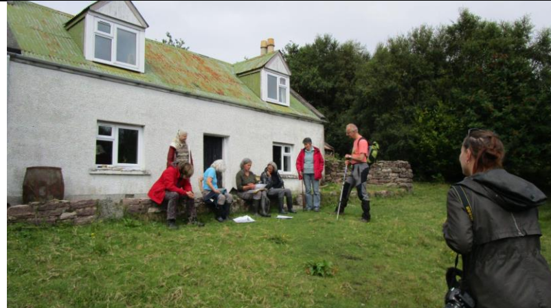
Original state of the building © Isle Martin Trust
