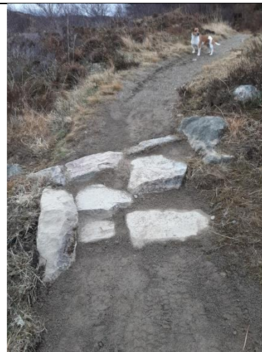
New steps and water bar at Little Assynt © Fiona Saywell/Culag Community Woodland Trust
