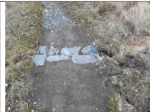
New steps and water bar at Little Assynt © Fiona Saywell/Culag Community Woodland Trust
