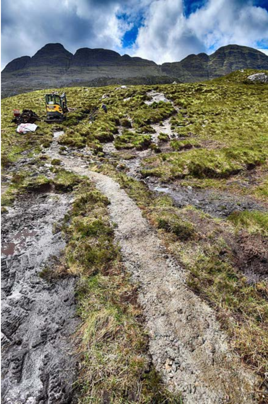
Above: The path work has an impact too but once the work is complete vegetation can begin to recover on the ground adjacent to the path. Photo © Chris Puddephatt.
