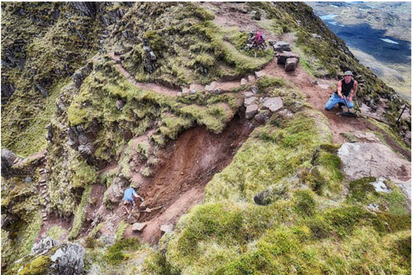
Johny winches stone down the badly eroded gully. Photo © Chris Puddephatt.
