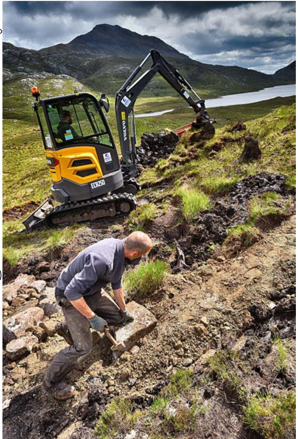
A.C.T. Heritage busy shifting materials to construct the path. Photo © Chris Puddephatt.
